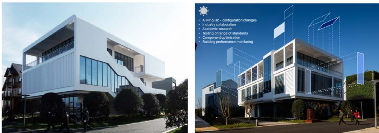
Figure 10. The P+ Demonstration Building: north –east corner with vertical gallery and external platforms and south-east corner with smart louver systems and ‘plug and play’ facades.
